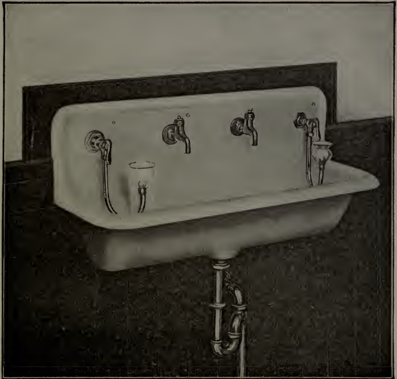
Type of sanitary drinking fountain installed in schools by placing bubbling-cups on old fixtures.
